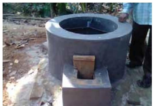
Mixing Device of Biogas plant
