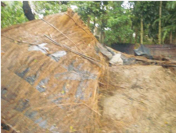
A devastated household after cyclone
