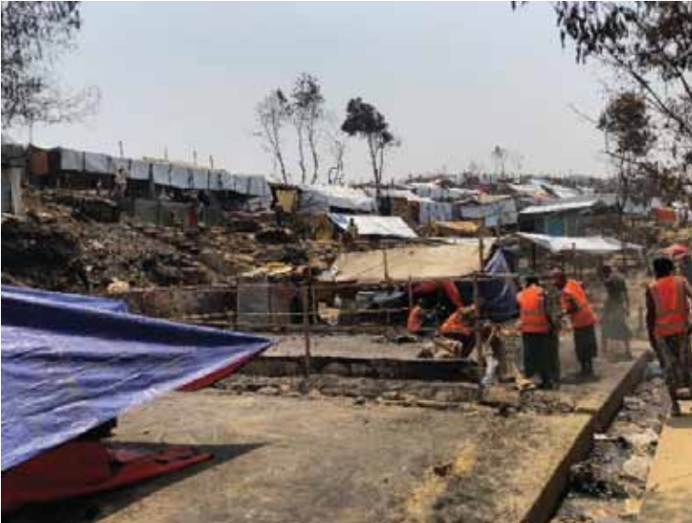
Volunteers are seen removing the debris
