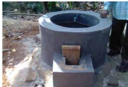
Mixing Device of Biogas plant
